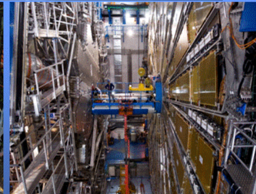
Installation of the last LHC beam pipe in ATLAS Detector
